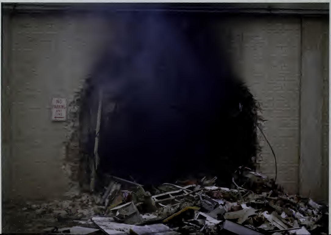
Above: In A-E Drive, debris and airplane tire remnant. Below: The “punch out” hole in A-E Drive.
